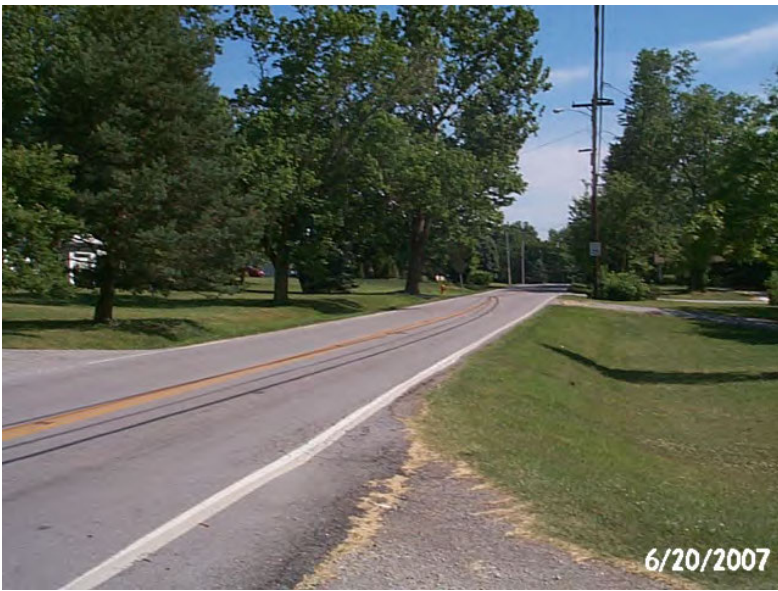
Photo 38 Gilliland Road South bound at Eastwood Cutoff
