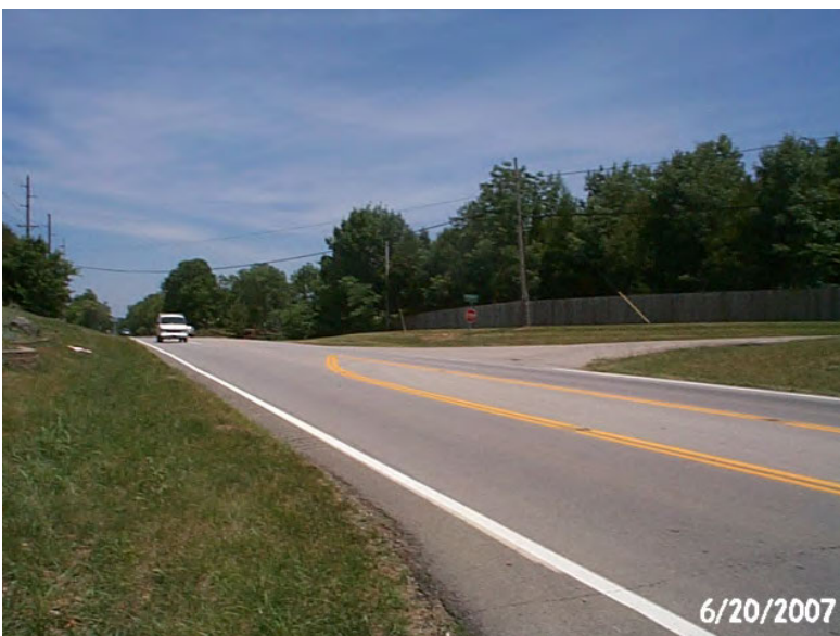
Photo 3 US 60 EB at Eastwood Cutoff
