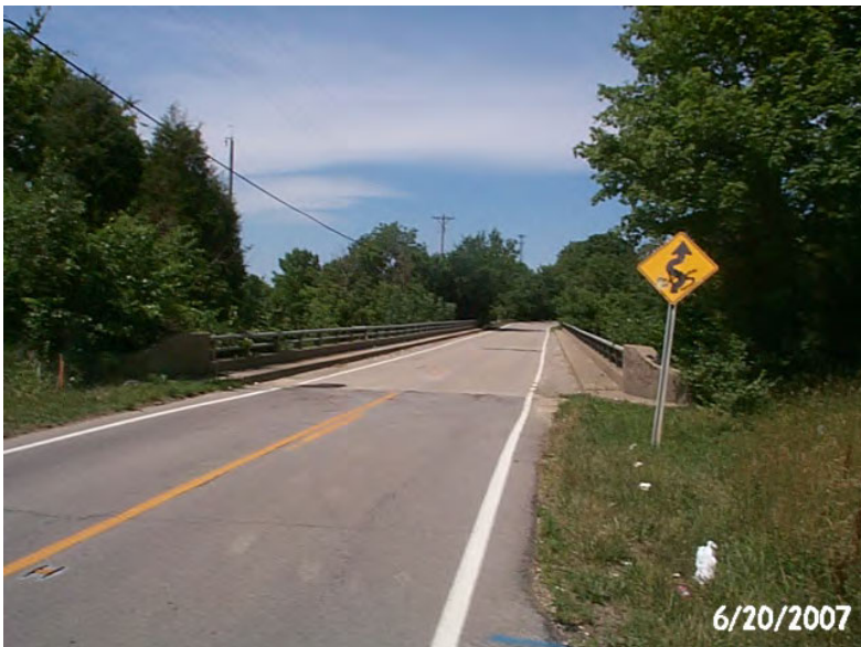
Photo 12 Gilliland Road North bound bridge over I-64
