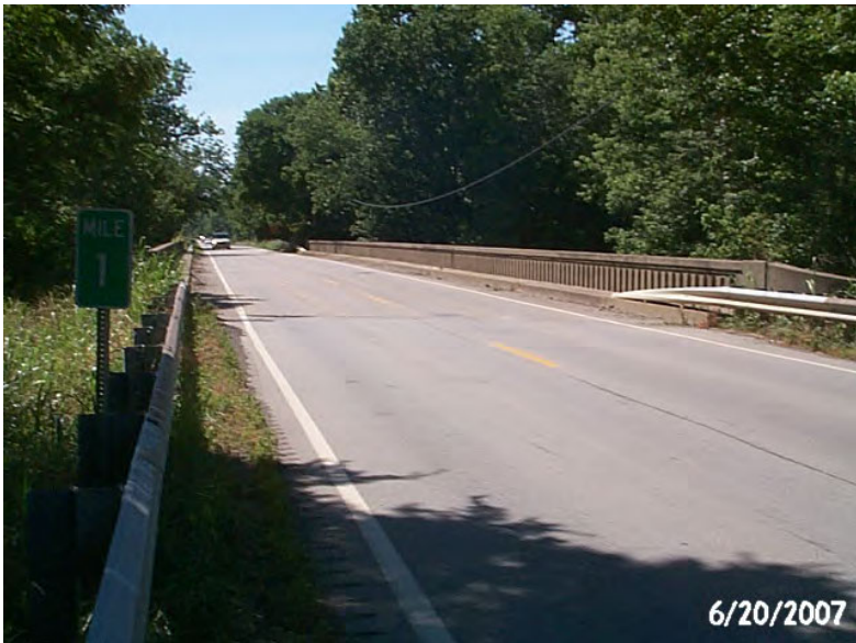
Photo 29 KY 148 West bound at Floyds Fork Bridge
